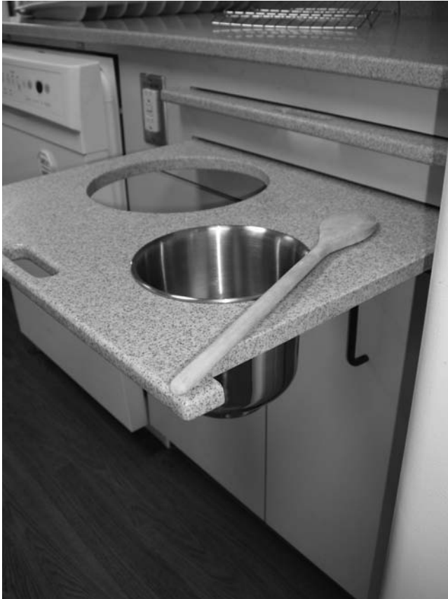
Figure 12-4 A pull-out shelf with cut-outs that accommodate bowls or pots enables a person to cook efficiently from a sitting position, e.g., when in a wheelchair.
